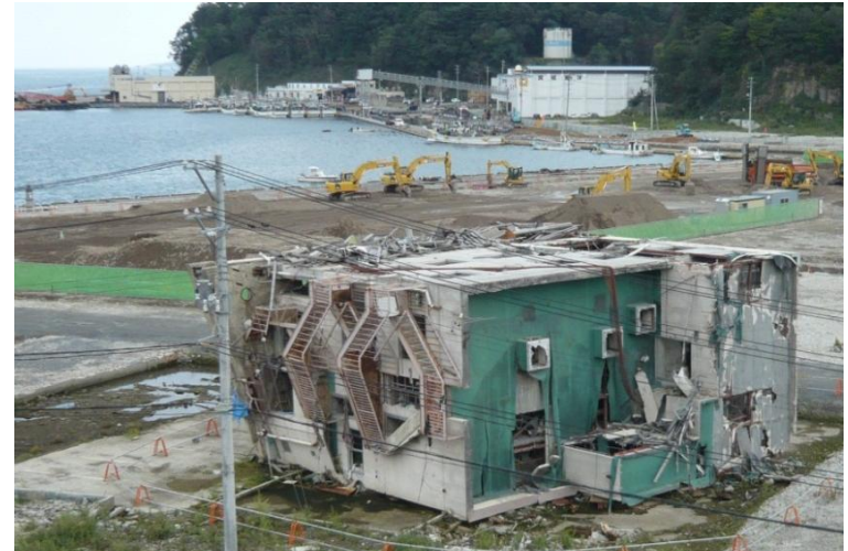
Building toppled by 311 tsunami
