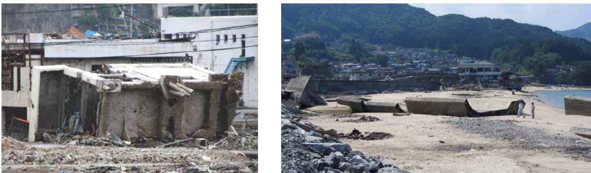
Figure 1 –RC building and seawall failures by overturning moment.
